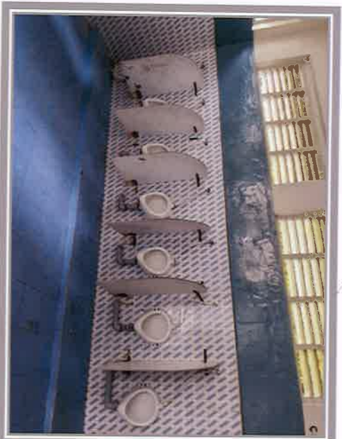
View of the Urinal
